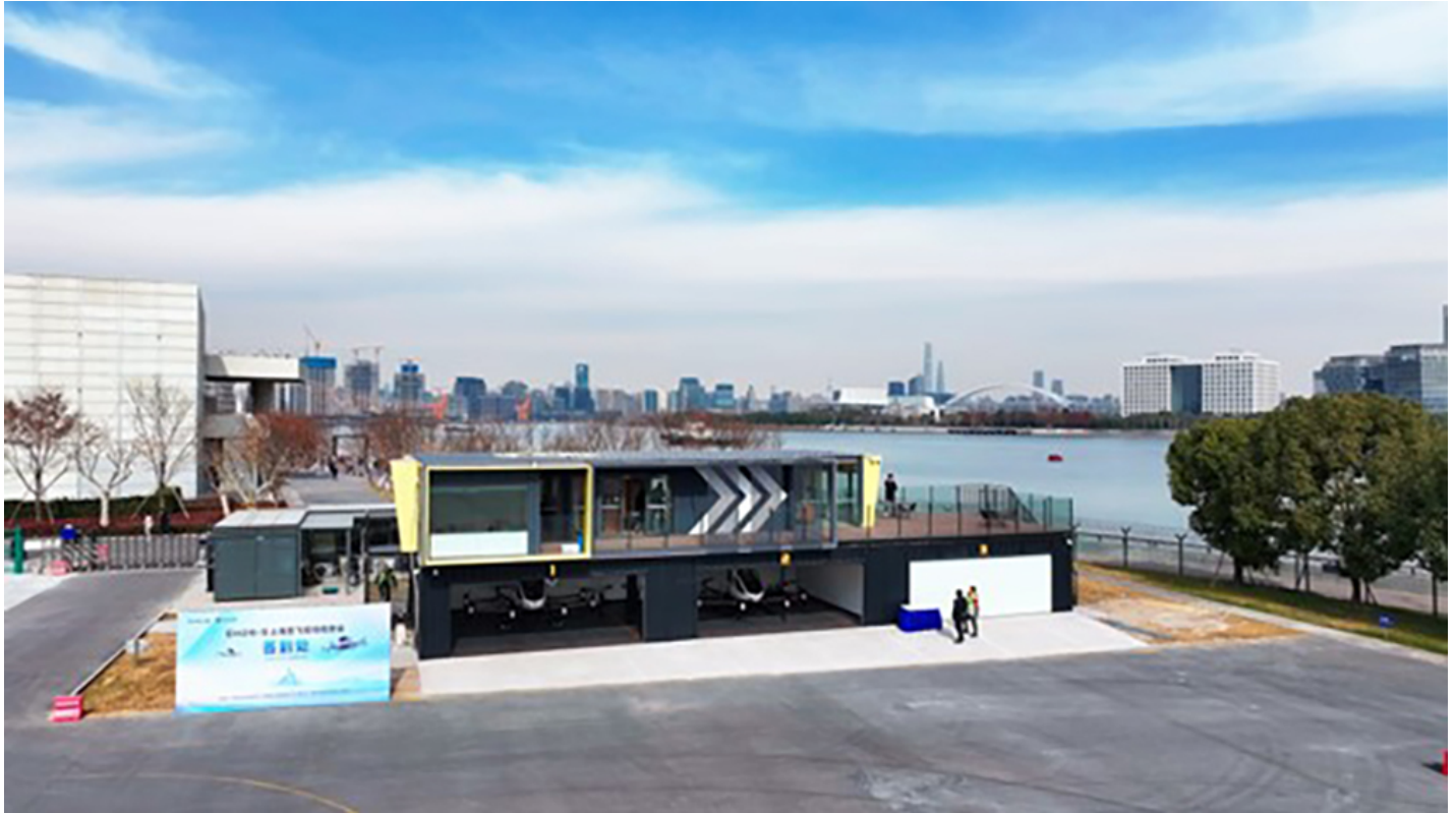
Image: EH216-S eVTOL operation center at Longhua Airport in Shanghai
