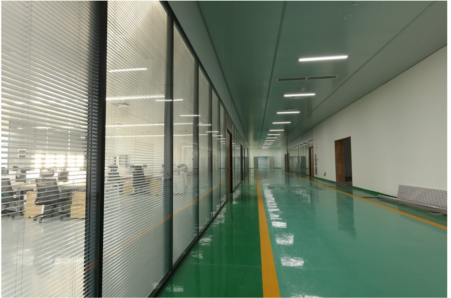
Office area of the EHang Yunfu facility
